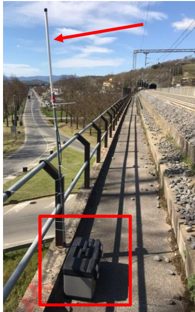
Figure 4 Base station box and its antenna.
