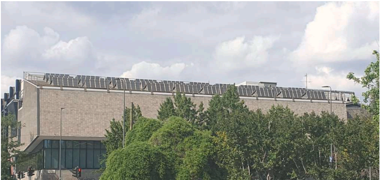
Fig. 2. Picture of the building 11 with the BIPV sheds.
