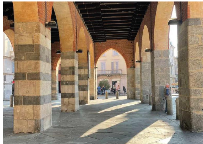
Figure 9. View of the columns NOPQ (on right) and GHIK (on left) (See Figure 7). The GHIK columns are built with alternate white and grey stone blocks, similar to the façade of the Monza Cathedral.
