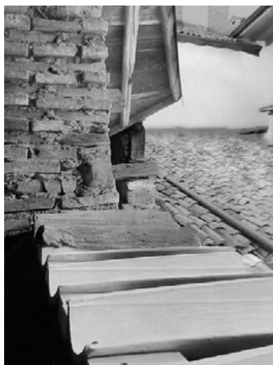
Figure 5. Above: the opaque part of the wall after completion. Below: views of the opaque wall cladding and of the sill on top of the wall "breach" [photos: Luca Panzeri and Noemi Riva, 2022].
