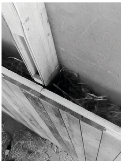
Figure 5. Above: the opaque part of the wall after completion. Below: views of the opaque wall cladding and of the sill on top of the wall "breach" [photos: Luca Panzeri and Noemi Riva, 2022].
