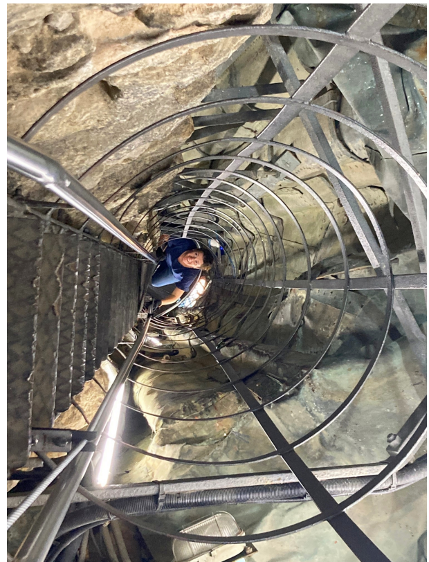
Figure 16: View of the internal vertical metal ladder equipped with safety hoops.
