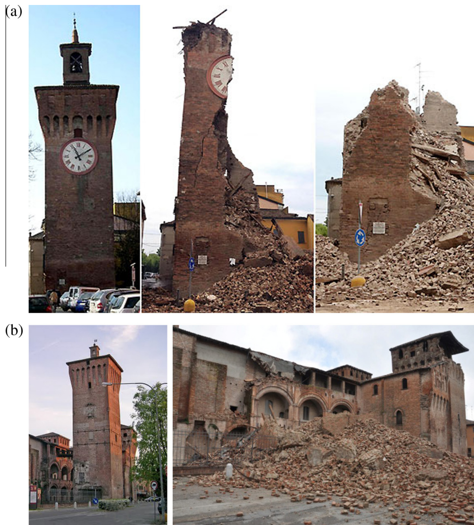
Fig. 2. Collapse sequence for the Clock Tower (a) and the Fortified Tower (b).
