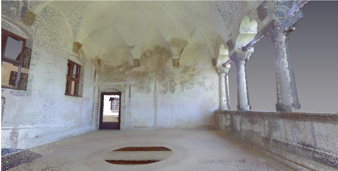
Fig. 39 Internal view of the loggia; high point density gives detailed representation of individual features.
