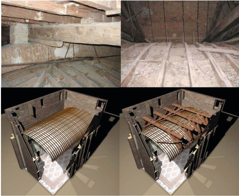
Fig. 12 Above, images of the extrados of the wooden vault of the Ballroom. Below, 3D model of the vault.
