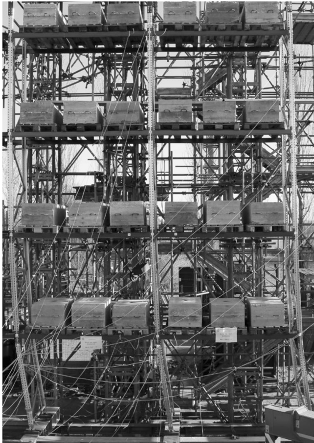
Fig. 19. Soft-storey mechanism formed at the first level.
