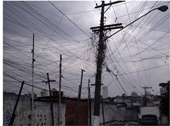
GIVE ELECTRICITY TO THE GRID
