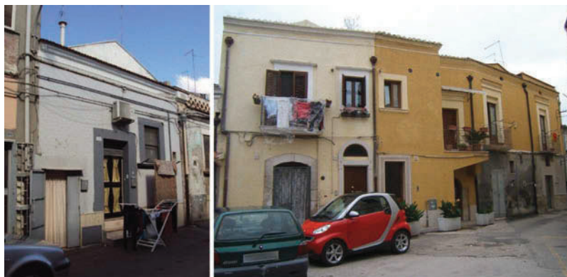
Figure 3. On the left, an example of the original configuration of the houses built after the 1731 earthquake. On the right, the same typology of houses after the addition of a story and an enlargement.
