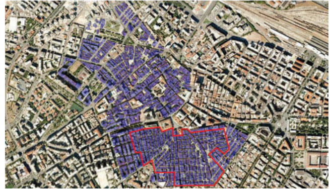
Figure 4. The historical center of Foggia, with the surveyed buildings in evidence. The area object of the reconstruction of 1731 is marked in red.
