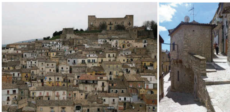
Figure 6. A view of Sant'Agata historical center (left), and an example of the typical structural aggregate, built on a slope with two level elevations (right).
