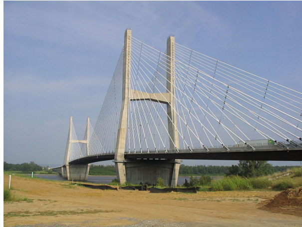
Fig. 17 The Bill Emerson Memorial Bridge (Framerotblues 2007; with permission)
