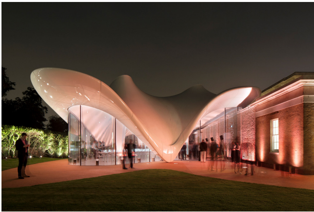
Fig. 1. Zaha Hadid Studio, Serpentine Sackler Gallery, London. Permanent building with double textile membranes roofing system integrated with glazing eyes on the top. (Copyright reproduced courtesy of Architen Landrell Associates.)
