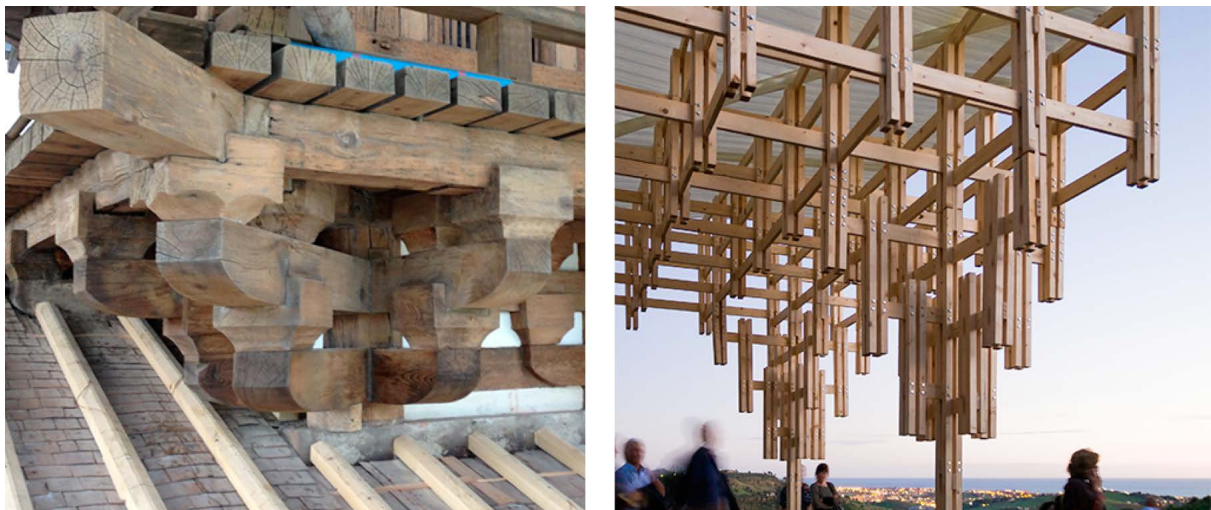
Fig. 7: The traditional Japanese bracket system and its reinterpretation.
