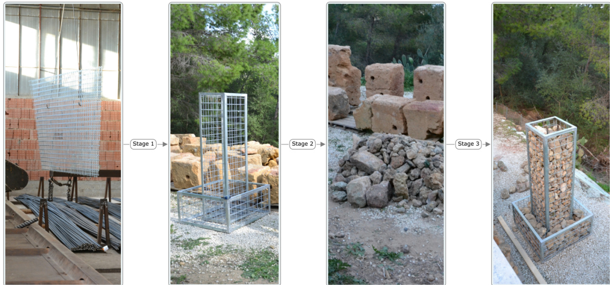
Fig. 4: Gabion walls during the construction stage of the AkragaShelter.
