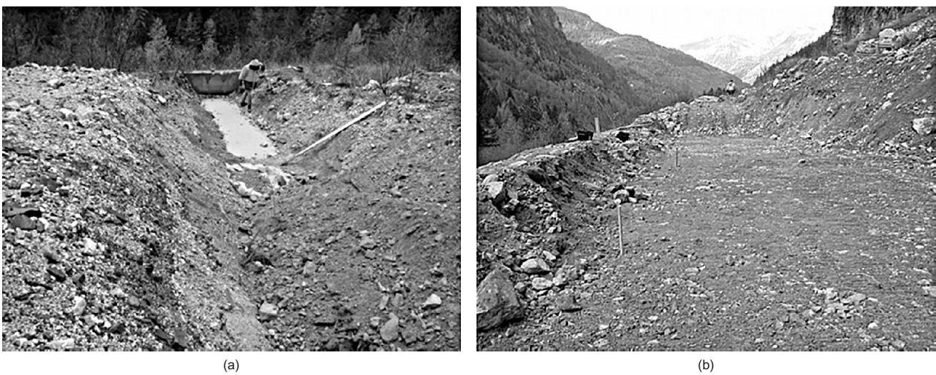
Fig. 4. Preparation of impact area: (a) trench excavation; (b) compacted impact area
