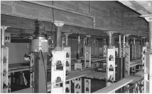
Figure 11. Prop and hydraulic jacks at beam No. 3.
