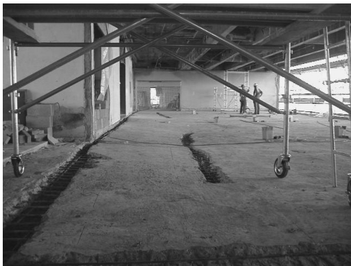
Figure 5. Yield lines after concrete demolition.
