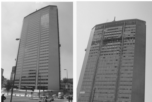
Figure 1. Pirelli building before and after the crash.
