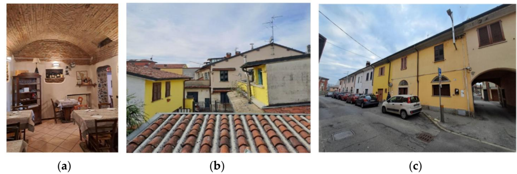
Figure 2. Example of recurrent residential masonry houses in the historic centres of Milan hinterland (in Paullo): (a) one with a brick masonry vault at ground floor; (b) simple buildings arranged around an open courtyard and (c) in a row along the street.
