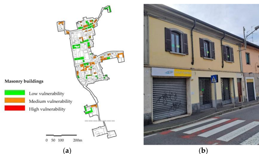
Figure 1. Milan hinterland (Paullo, Italy): (a) fast and non-invasive investigation method for the acquisition of a picture of the overall level of vulnerability of the residential built heritage of a city; elaborated from [15]; (b) example of masonry buildings with the insertion of large openings on the ground floor.
