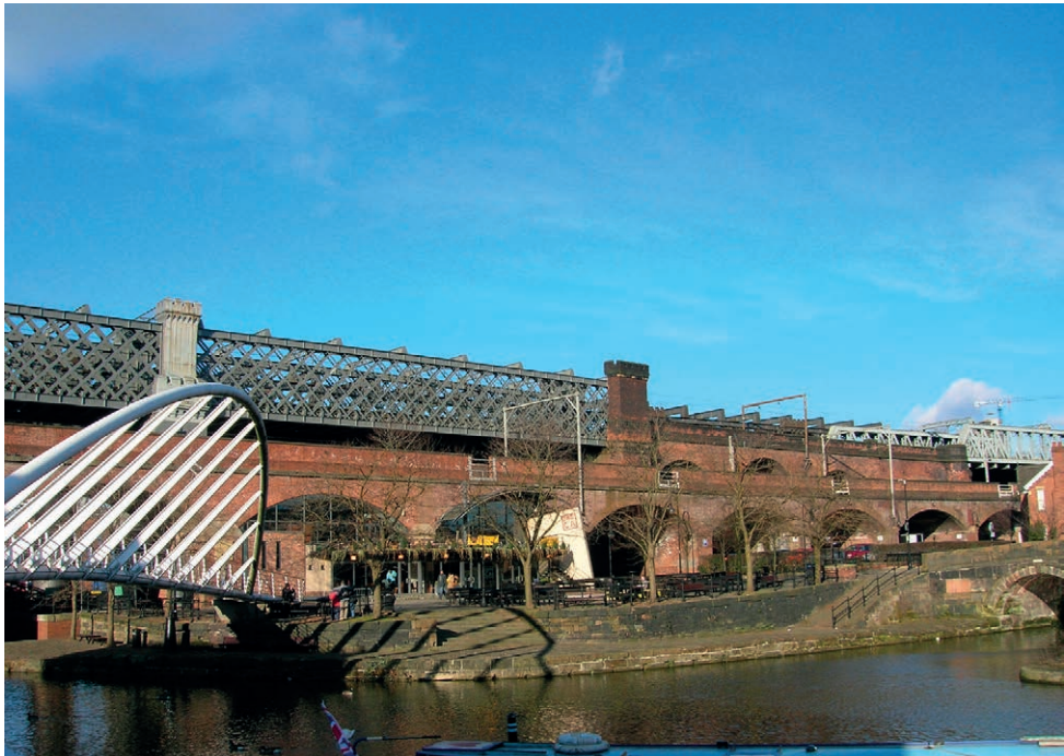
Figure 2 - Castlefield Conservation Area, near university campuses in Manchester (photo by Cu- turi C., 2006).
