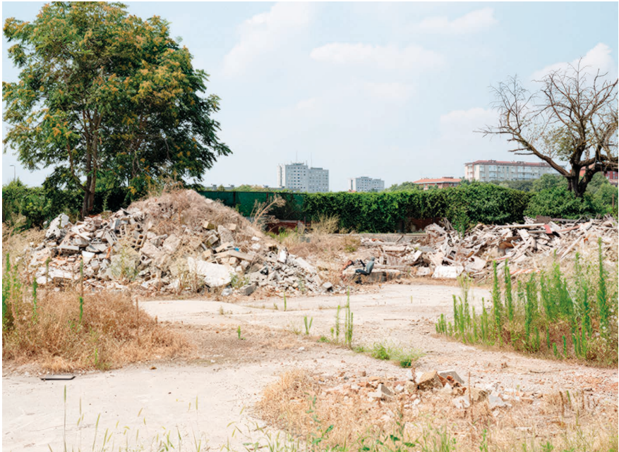
↑ Piles of demolition rubble in the project site.
