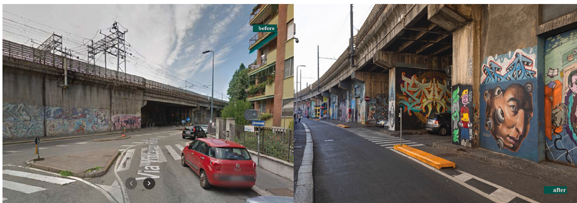
Fig. 4. Project 3: the intersection of via Pontanto/via Morandi before and after the intervention (Comune di Milano, 2023).
