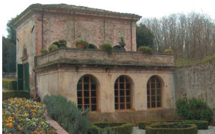
Figure 5: Southwestern view of the coffeehouse
