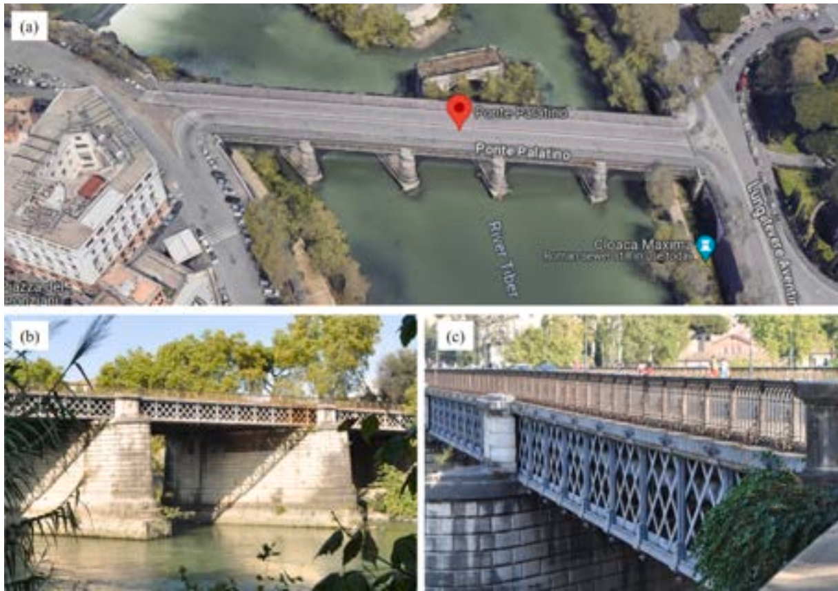
Fig. 7. Palatino bridge: (a) Aerial view of the bridge (from Google Maps); (b) Focus on the piers; (c) Focus on the continuous beams.
