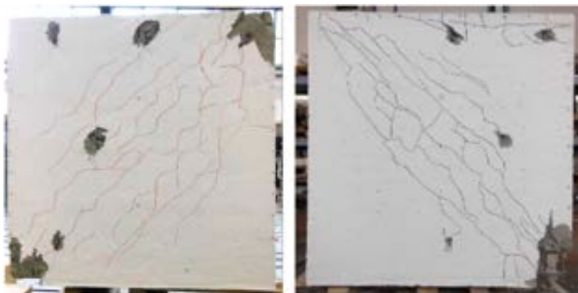
Fig. 8. Damage pattern at the end of the test for specimens MR2-3-8-C-1 and MR2-5-8-C-2.
