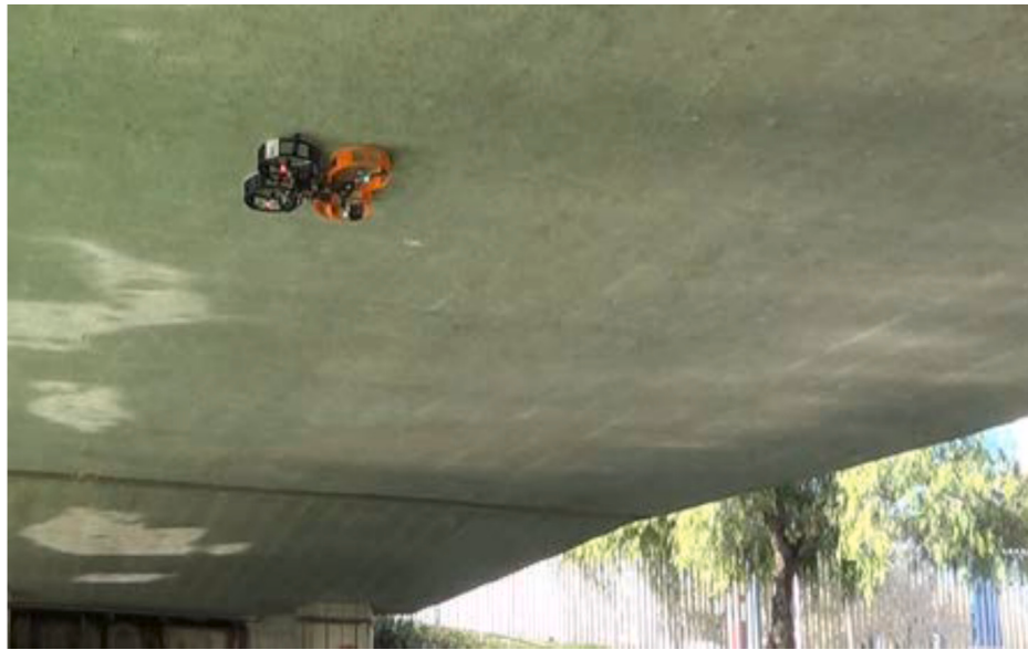
Fig. 9. Drone hovering attached to bridge intrados [114].
