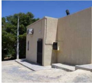
Water Quality Control Laboratory
