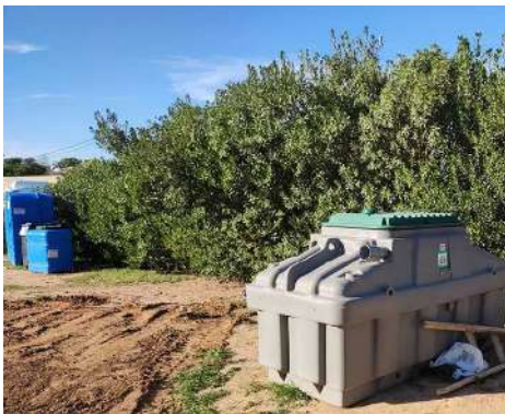
Ecoflo biofilter for domestic wastewater treatment
