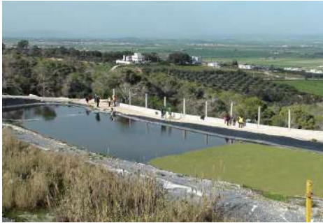
Sidi Amor wastewater reuse pilot basin
