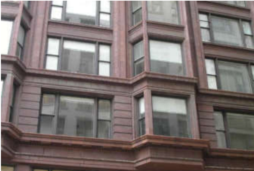
Fig. 1.24: Holabird & Roche, Marquette Building, Chicago, 1895.
