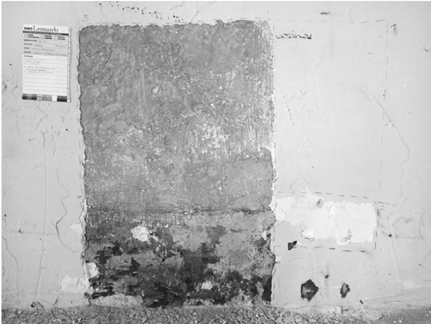
Fig. 6 The bichrome area between the beige wall and the brown plinth, visible in the lower areas of the walls of Hall C and the pillars of Hall B
