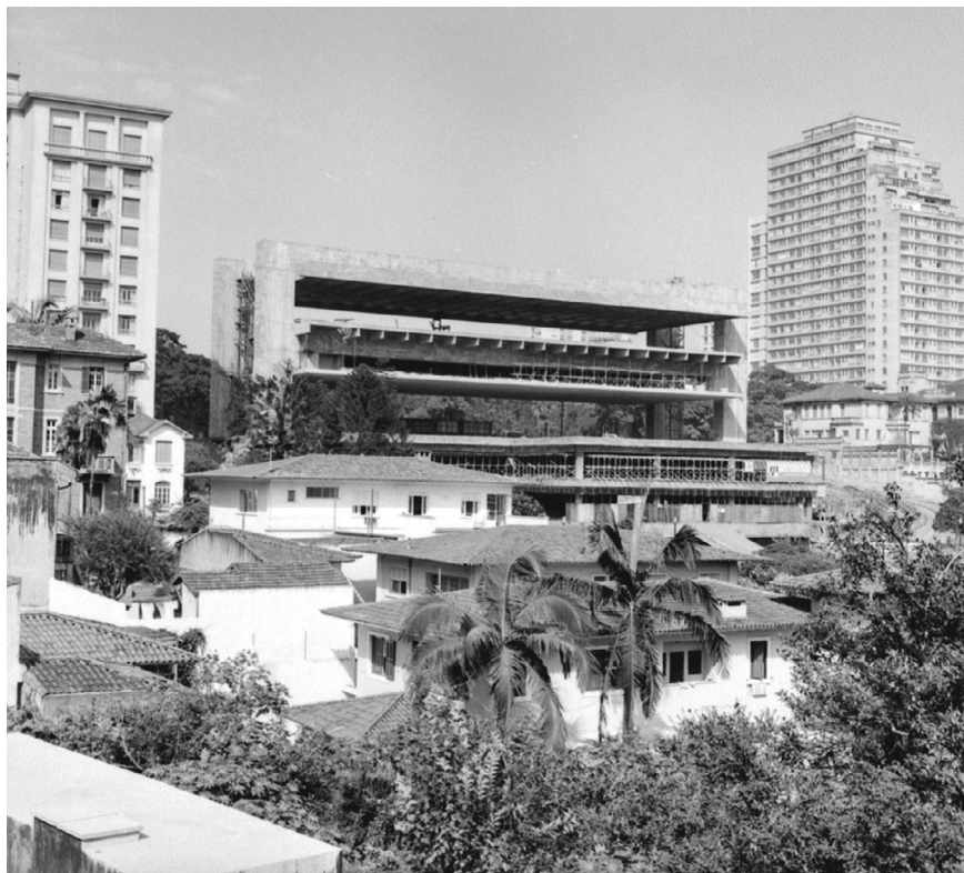
Fig. 4 The MASP under construction https://www.getty.edu/foundation/initiatives/current/keeping_it_modern/report_library/masp.html
