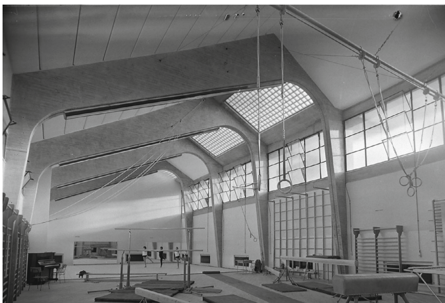
Fig. 2 The Stadio Flaminio gym under the west grandstand (ICCD Archive)
