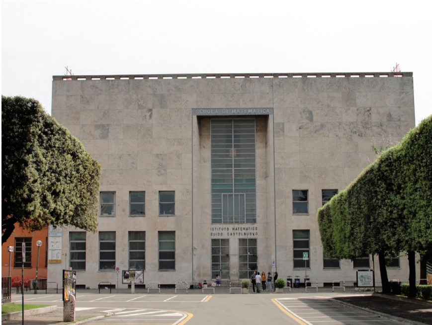
Fig. 1 The School of Mathematics at Rome's university campus, front building (photo N. Sardo)
