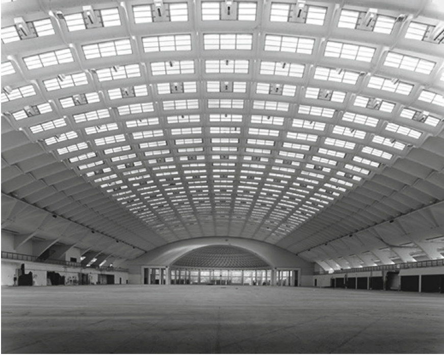
Fig. 5 Hall B, after the clearing and cleaning operations for the execution of the tests within the Keeping It Modern project (courtesy of Fabio Oggero, 2022)
