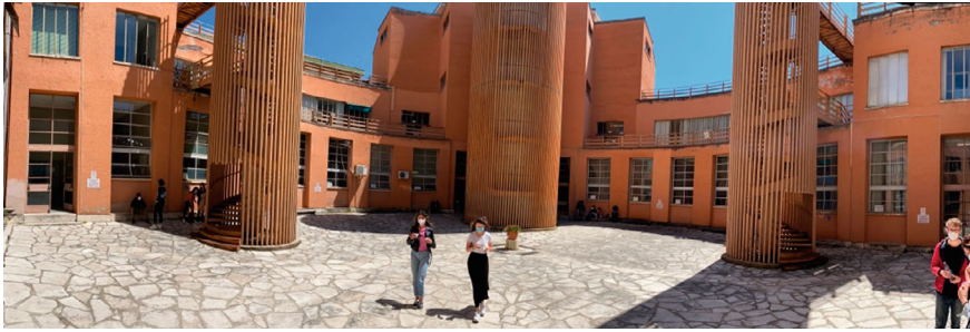
Fig. 5 The fire-escape staircases placed in the courtyard in the eighties (photo Salvo, 2021)
