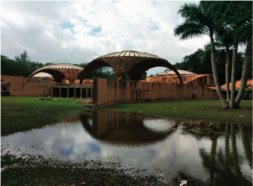
Fig. 6 Ballet School flooding, January 2019, photo by Davide Del Curto
