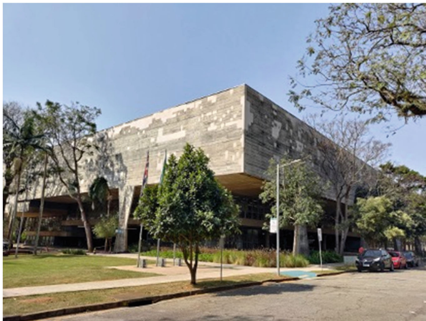
Fig. 5 Vilanova Artigas building: façades after works, 2023 (Photo Beatriz Kühn)
