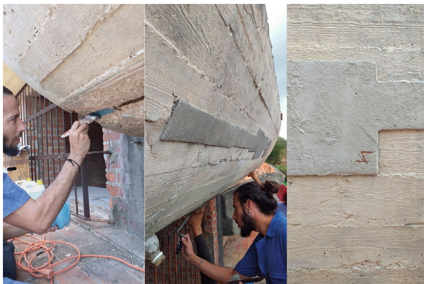
Fig. 5 Pilot site for reinforced concrete's restoration. Courtesy of Assorestauro, photo by Davide Del Curto
