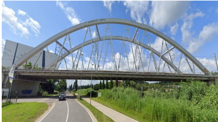
Fig. 1. The KW51 Bridge
