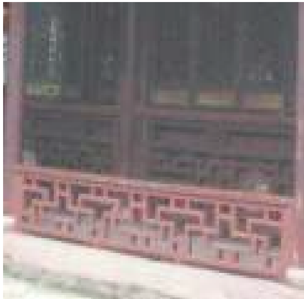
Fig.64 Wood Handrail in SuZhou ZhuoZheng Garden
