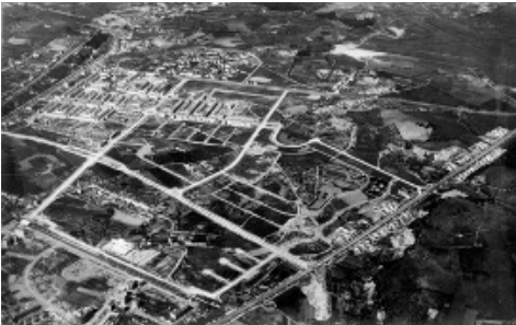
Fig. 5. Unknown author, Aerial view of the Alvalade infra-structures works underway, in the rural setting, 1950, Lisboa, Arquivo Municipal de Lisboa – Fotográfico . We can see the priority given to the social housing urban cells 1 and 2, already built (in the middle-left side), the commercial area along Av. da Igreja and cell 3, the Hospital Julio de Matos, and the private detached houses along the already completed Airport Avenue (diagonal, from bottom to right, overpassing the Sintra train line, and ending at the Airport Roundabout).
