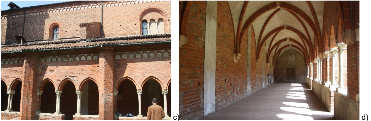
Figure 2. The northern and southern buttresses of Chiaravalle church: a) the external northern buttresses differently coloured according to their role: main one for the nave in red and the minor for the north aisle in pink; b) view of the northern buttresses from the lantern tower; c) the external southern buttresses, visible only above the aisle roof; d) the southern courtyard, where no buttresses are visible along the church wall on the left.
