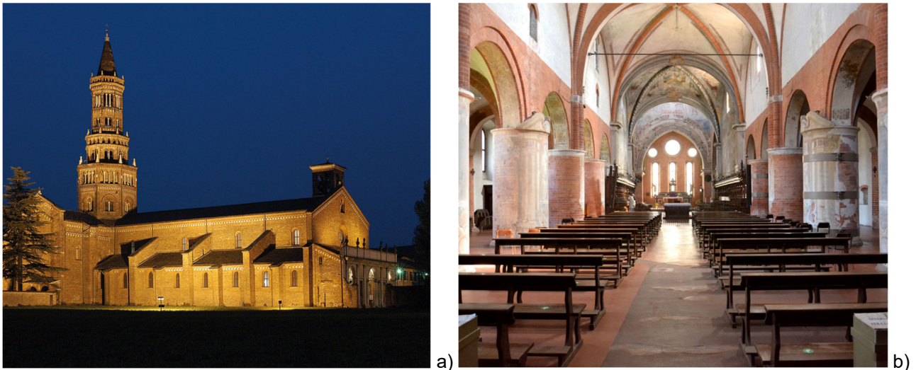
Figure 1. Chiaravalle abbey in Milan: a) view of the external northern side and b) view of the interior of the church with the difference in height of the three naves.
