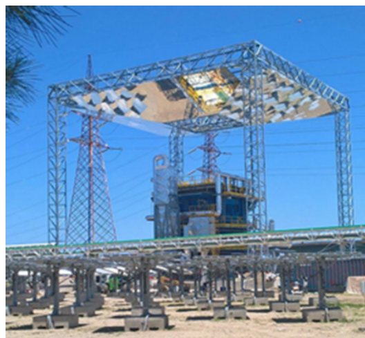
Figure 1. Magaldi STEM ® pilot plant in San Filippo del Mela, Italy.
