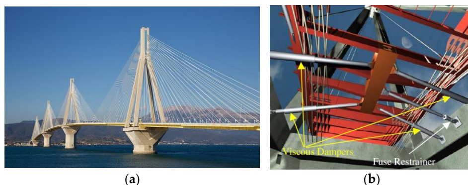
Figure 9. (a) The Rion-Antirion Bridge; (b) the seismic protection system of the suspended bridge [93].
