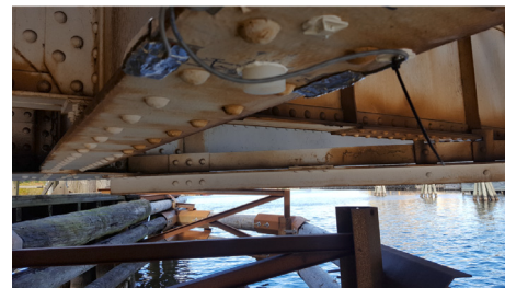
(b) Strain gauges placed at bottom flanges of the main crossbeams.
