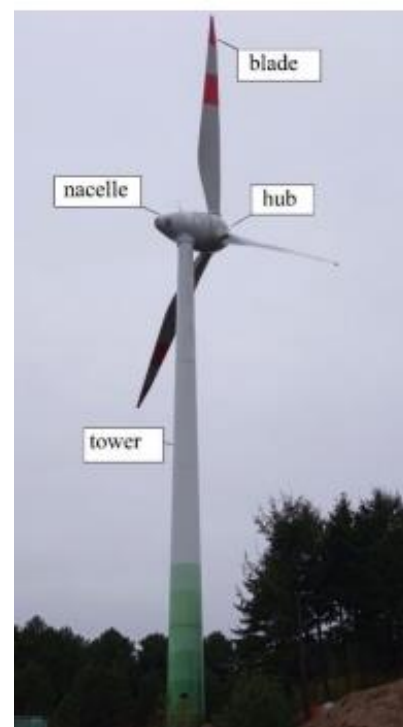
Figure 1 Tubular steel tower and its main components (courtesy of SEVA srl)
