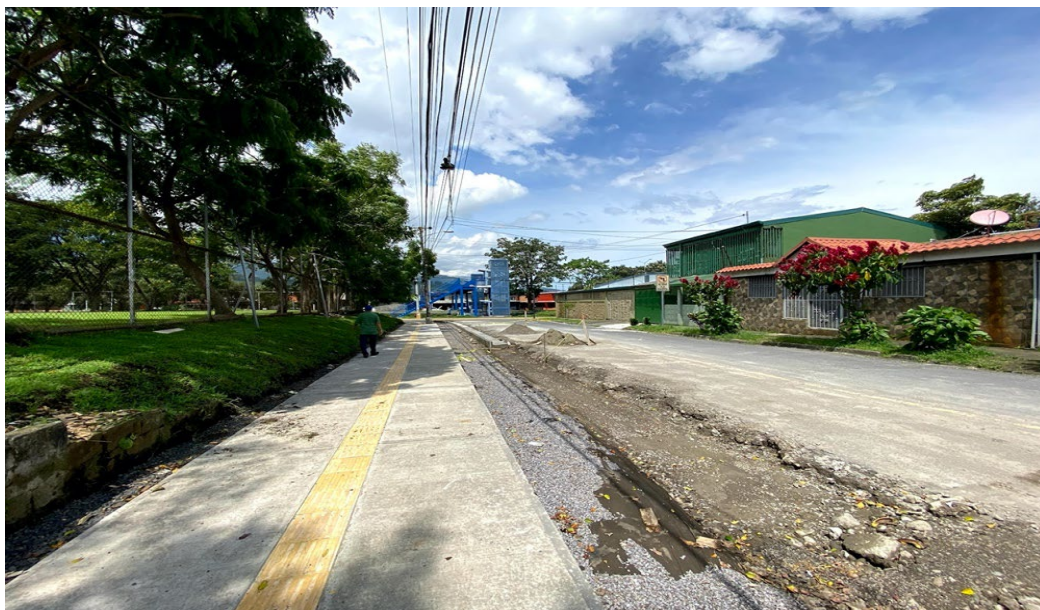
Figure 4. Nature Based Solutions (NBS) Intervention: Porous concrete sidewalk, Hatillo, San José, Costa Rica
