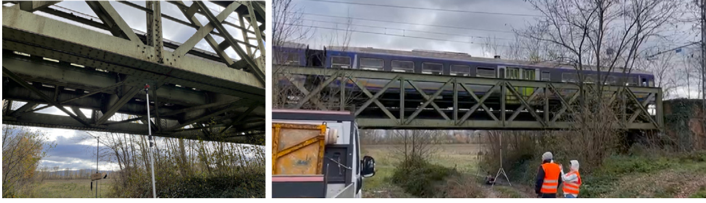
Fig. 10. Experimental setup; (b) View of the bridge under a two-cars train transit moving at 30 km/h.
