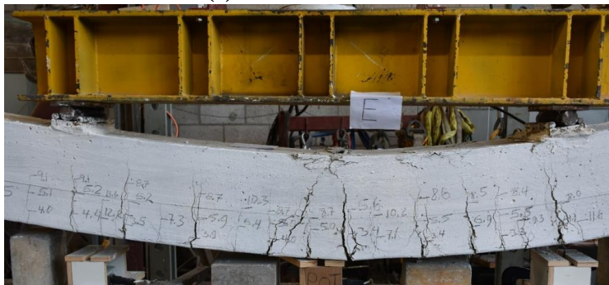
(c) Most cracks are wide
