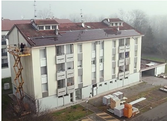
Figure 1. Case study residential building, Bagnolo, Italy
