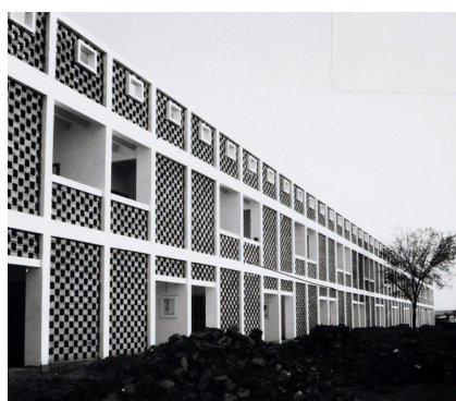
Figure 11. Mughal Jali in the Diwan-i Khas comparison with House Type 10-JB, Sector 22, Chandigarh, India. © Fondos Pierre Jeanneret colección Canadian Centre for Architecture, Montreal; Courtesy of Jacqueline Jeanneret
