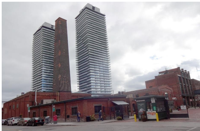
Figure 7. Old industrial sites transformed in the city of Toronto
