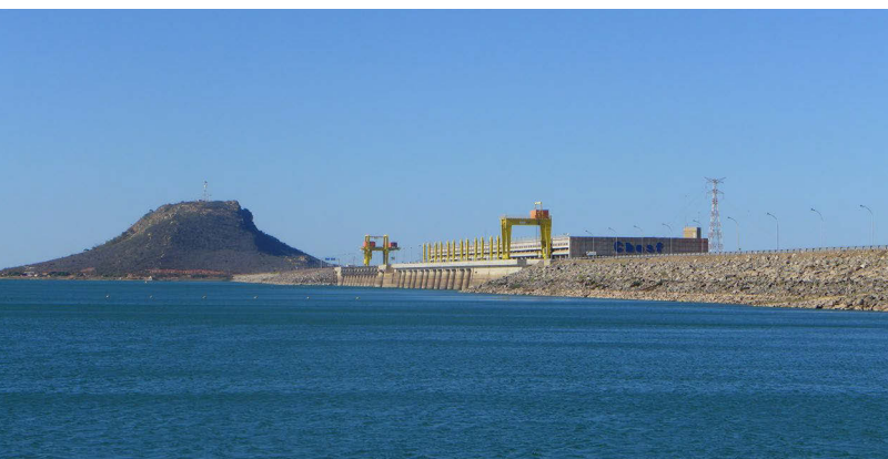
The dam and hydroelectric power station of the Sobradinho Reservoir. Photo: H Koch
