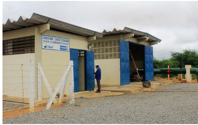
“EB5” pumping station infrastructure. Photo: W Souza
