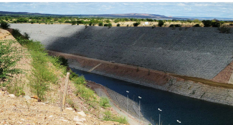
The channel that brings water from the Itaparica Reservoir to the first pumping station of the water diversion project (eastern channel system).
