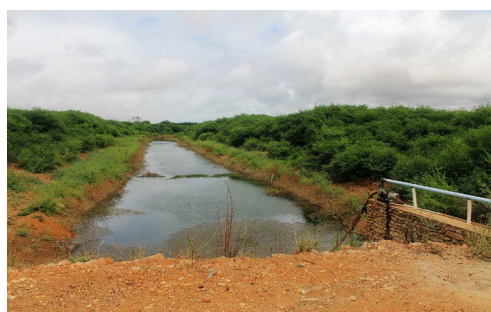
“EB5” pumping station channel. Photo: W Souza
