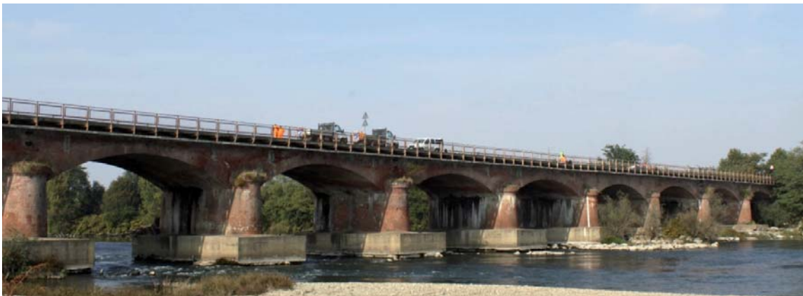
Fig. 1. The Candia bridge: view from the downstream of Sesia River.
