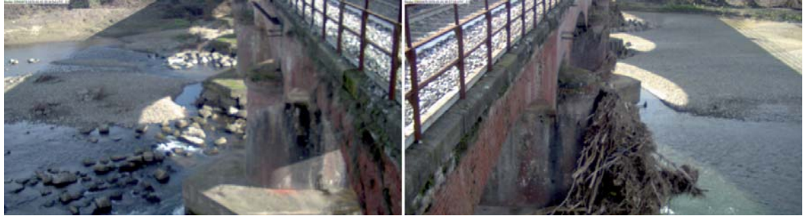
Fig. 4. Pictures of the upstream side from the permanently installed cameras.
