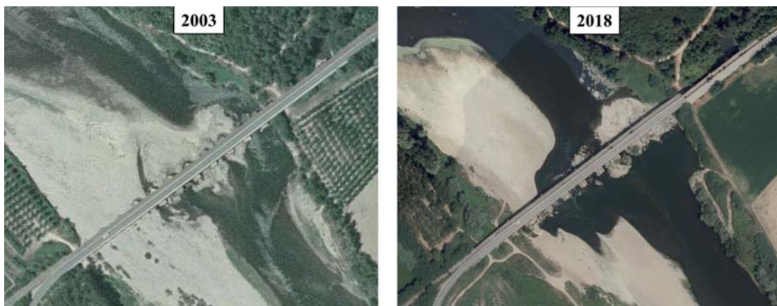
Fig. 2. Satellite images of the Sesia River before and after the armoring intervention.
