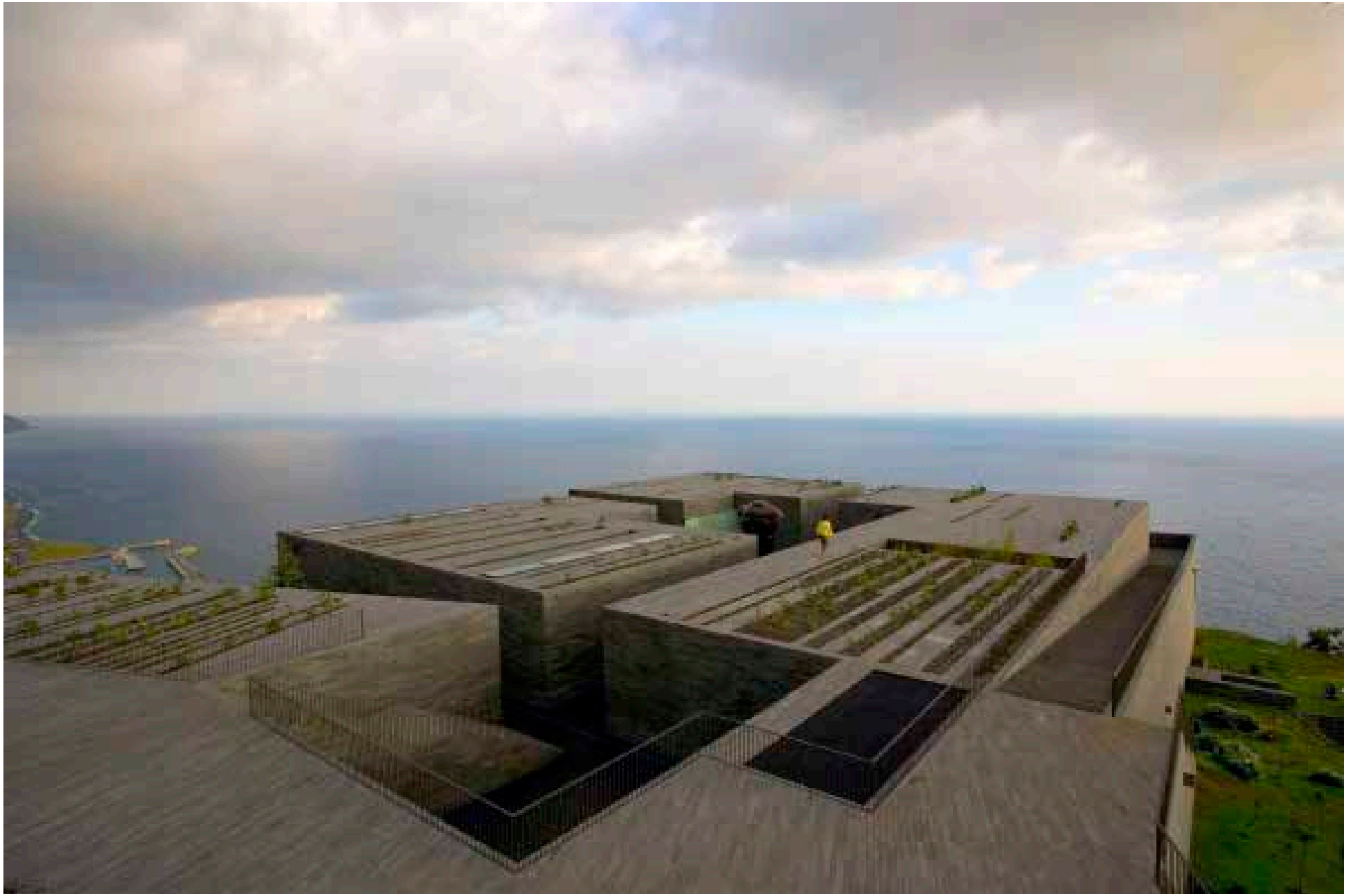
5 View of the roof level © Paulo David Arquitecto, ph. Fernando Guerra.
