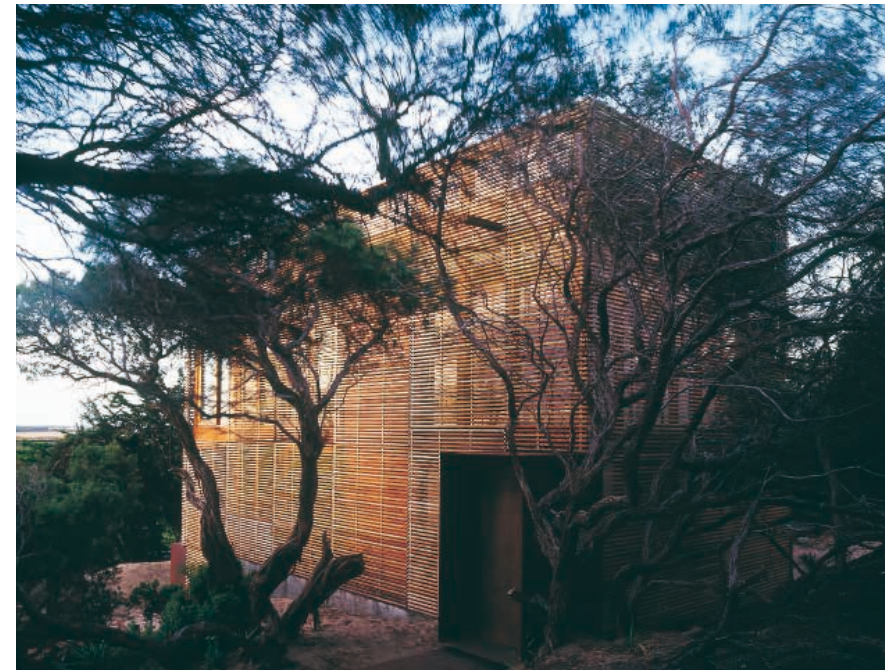
3 4 Exterior view of the Eastern and of the South-Western façades © Sean Godsell Architects.
