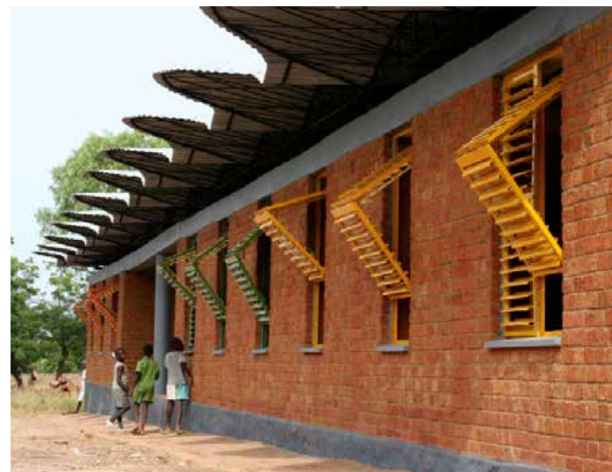
17 Overview of the building © Kéré Architecture, ph. Erik-Jan Ouwerkerk.
