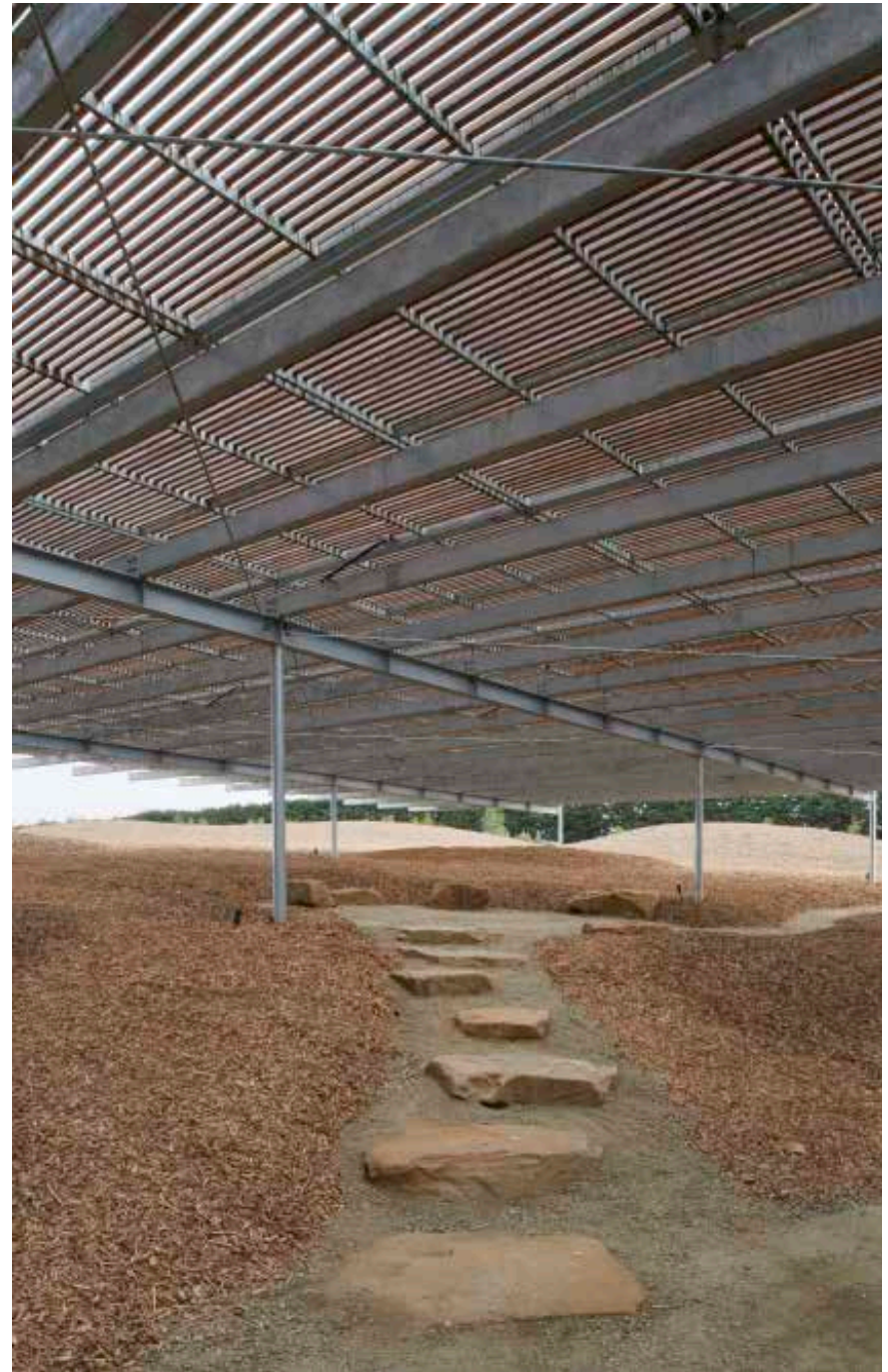
18 The protected outdoor space © Sean Godsell Architects.
