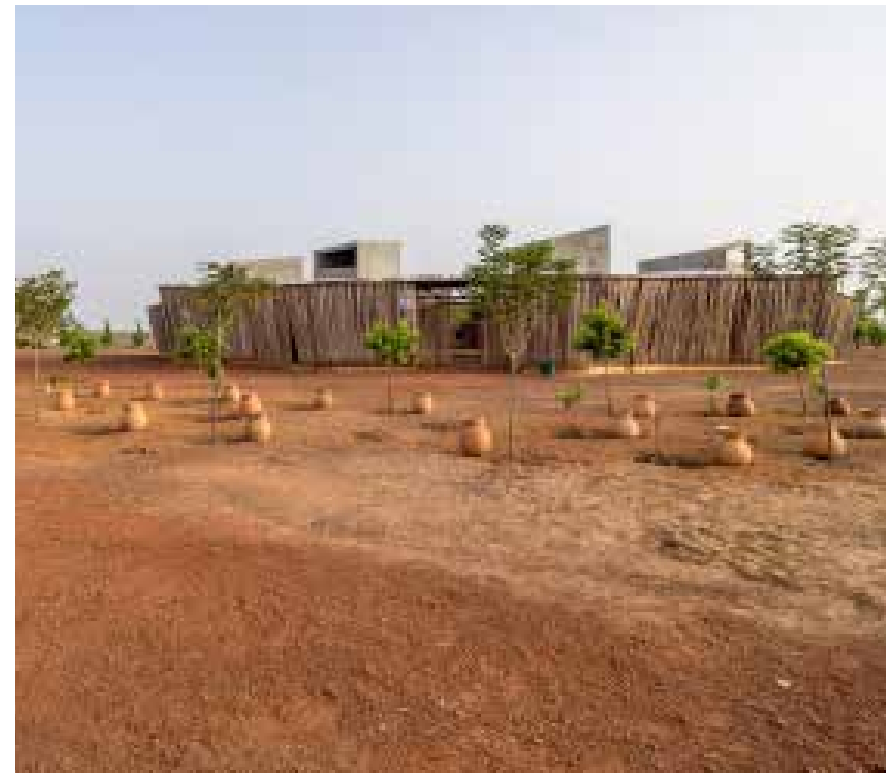
2 Detail of the façade @ Kéré Architecture.
