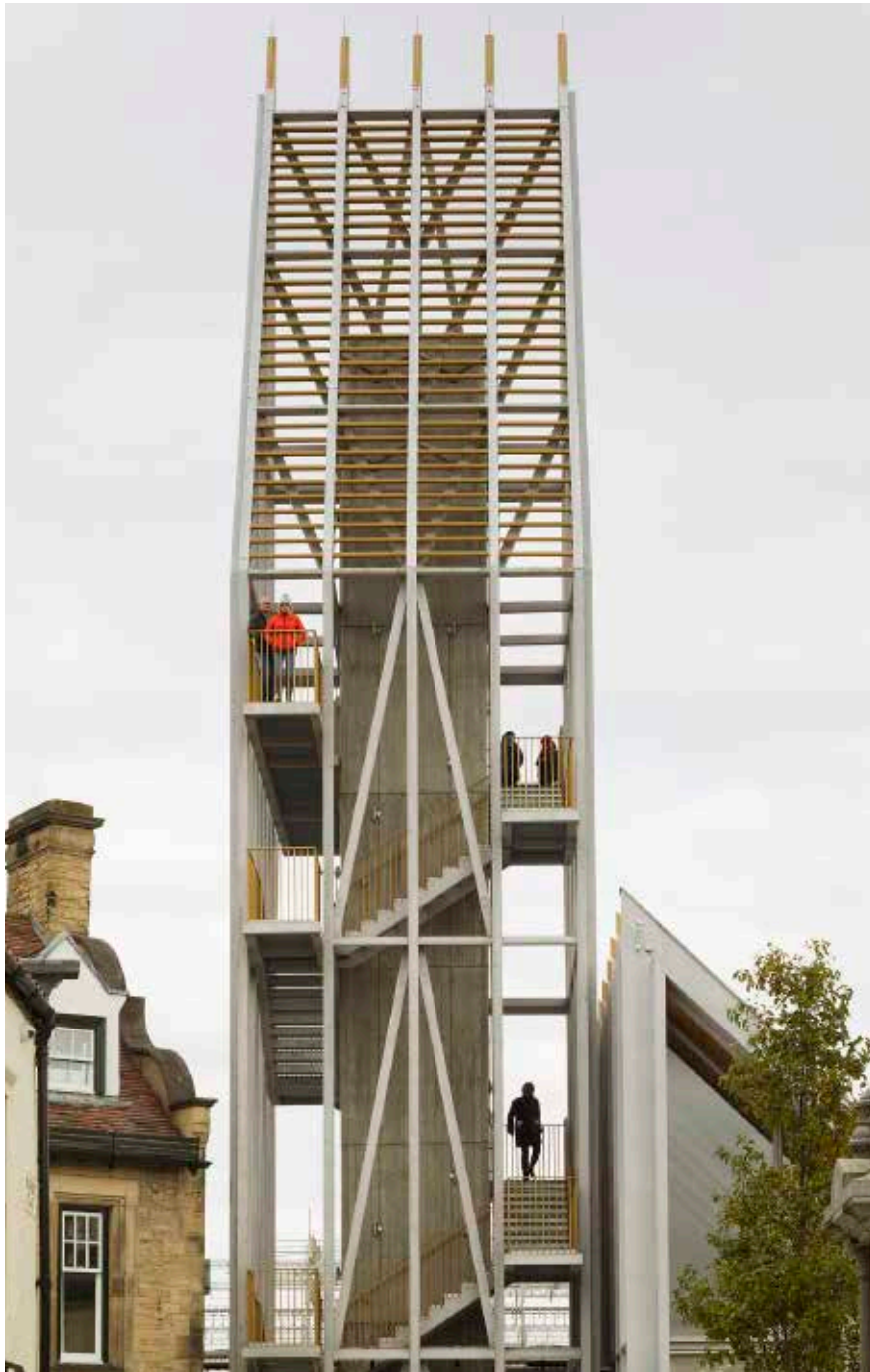
14 The Tower © Niall McLaughlin Architects.
