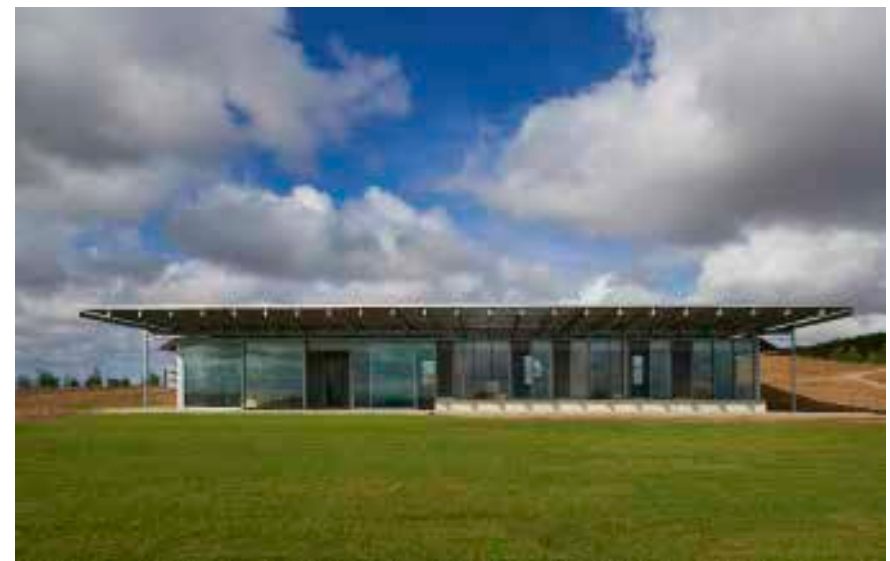
13 14 15 The roof screens, closed and open, and the exterior view © Sean Godsell Architects.
