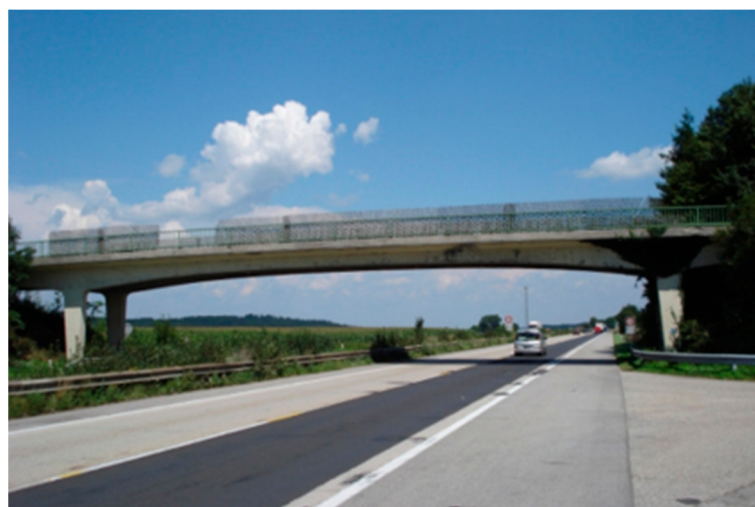
Figure 7. S101 bridge—West side [29].
