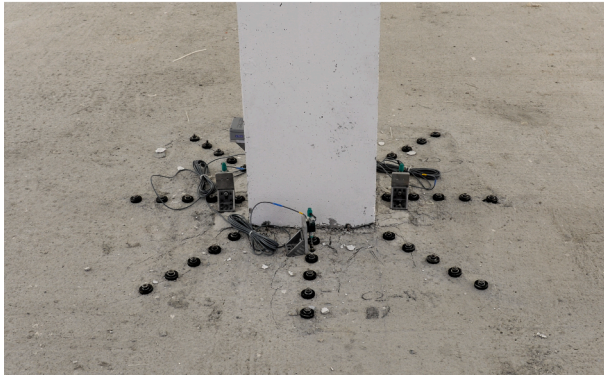
(b) Strengthened interior slab-column connection C2-1
