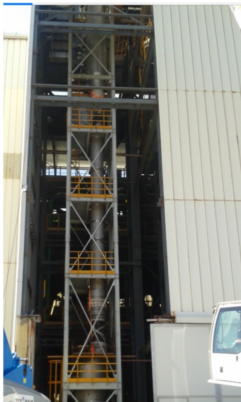
FIG. 31. Picture of the Seruci-0 column fully constructed and ready for the first tests.
