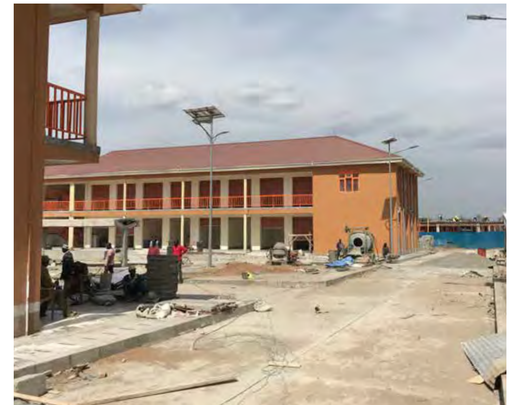
Arua Taxi Park under construction, 2018
