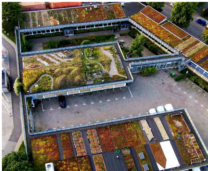
Fig. 4 – Giardino botanico in copertura di Augustenborg / Augustenborg botanical roof garden. (Source: http://scandinavian-green-roof.org/about/ourinstitute/ ).
