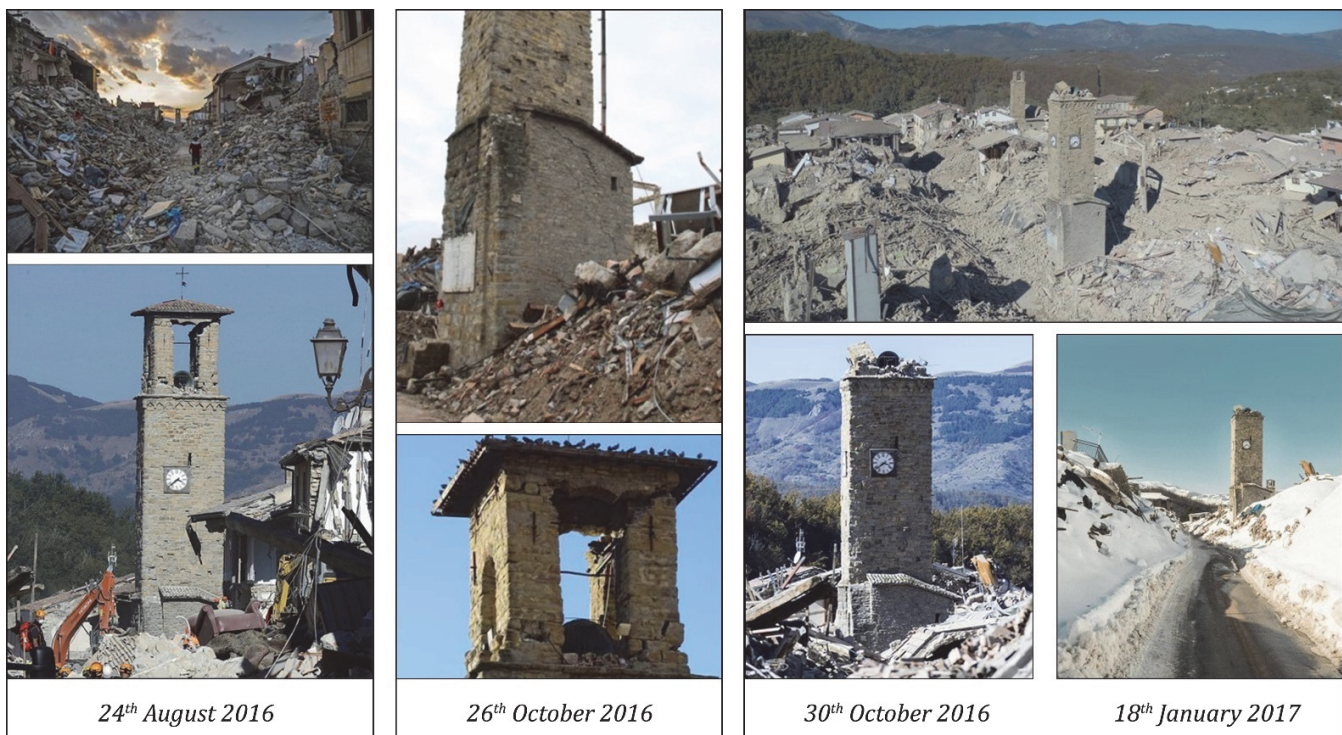
Figure 6: Views of the damaged civic clock tower of Amatrice (Rieti, Italy) after the main shocks of the Central Italy seismic sequence of 2016.
