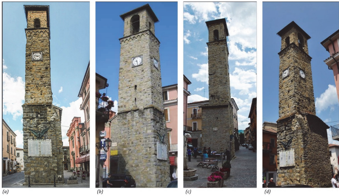
Figure 4: Views of the façades of the civic clock tower of Amatrice (Rieti, Italy) before the Central Italy seismic sequence of 2016
