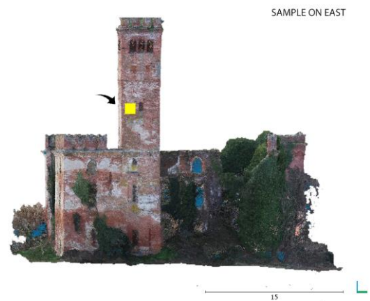
Fig. 6 Sample on East façade
